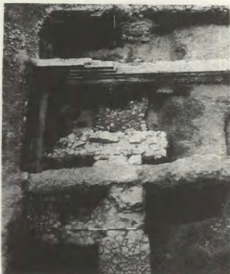
Pl 13 Bedford Castle: area E: BC72 55, south curtain wall, facing west.
